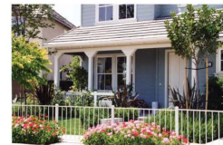
Porches are a dominant feature at streetscape
